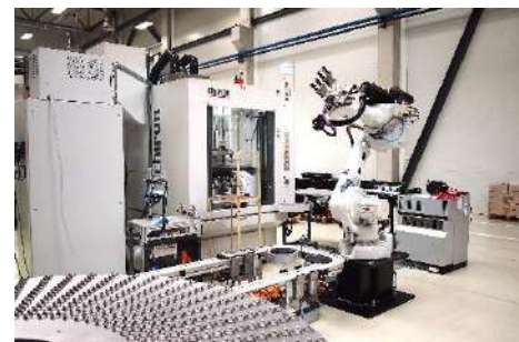
Extension of the processing line for the Pump Body, client Borg Warner
